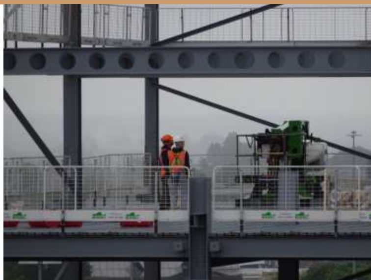
Council offices at Friargate under construction
